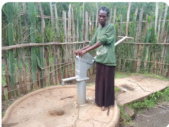
A rehabilitated hand pump in Aleta Chuko Woreda. WASHCO members operate the pumps on a fixed daily schedule and supervise their use.
